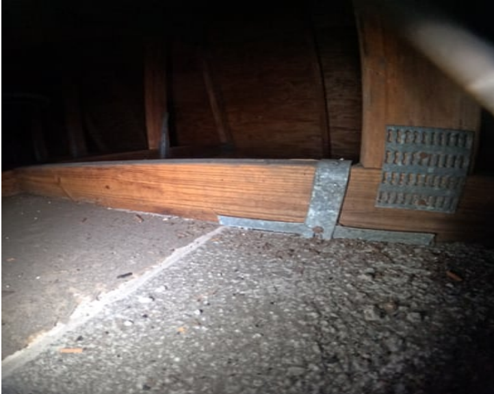
#3 toe nail 1 nail and 1 rivet front side
