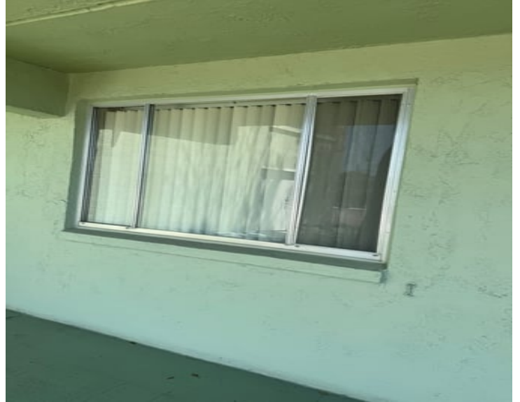
Stories 1-3 - Common Areas: Glazed (Protection Level-X) hoa office has 2 glazed openings
