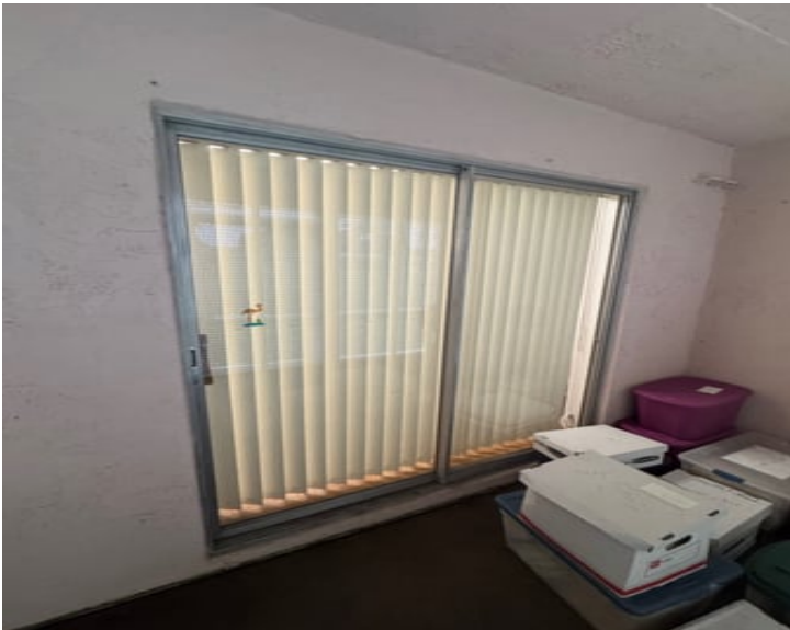
Stories 1-3 - Common Areas: Glazed (Protection Level-X)- hoa office
