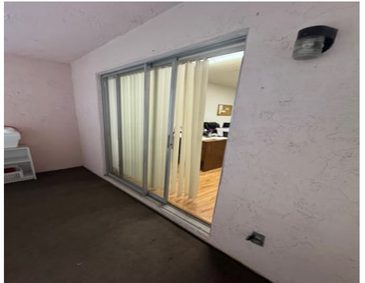
Stories 1-3 - Common Areas: Glazed (Protection Level-X)- hoa office
