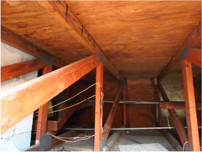
VIEW OF ROOF FRAMING
