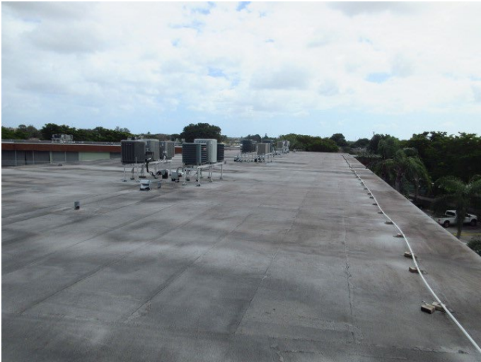
GENERAL VIEW OF ROOF COVERING
