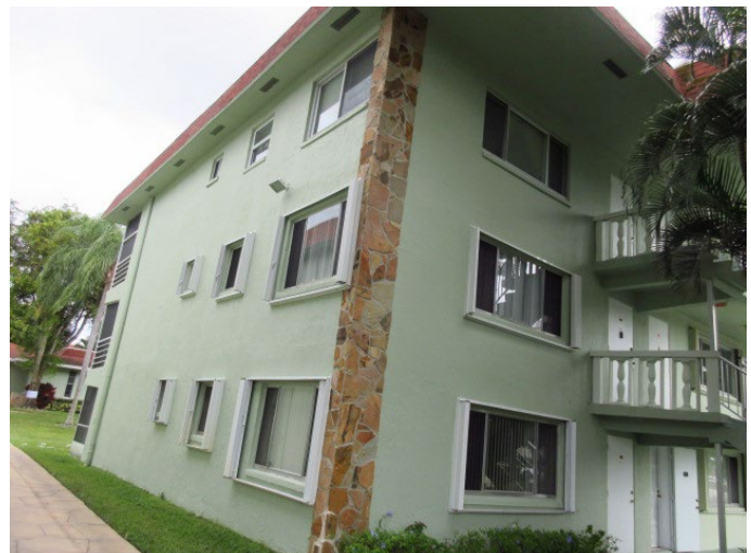
GENERAL VIEW OF BUILDING EXTERIOR FINISHES
