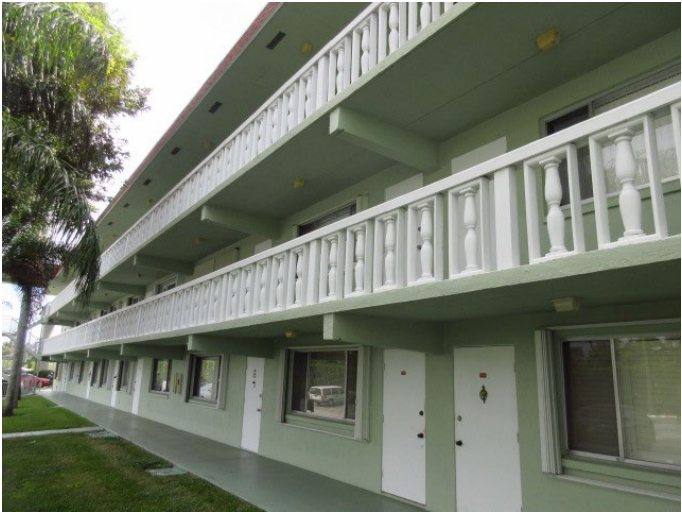
GENERAL VIEW OF BUILDING EXTERIOR FINISHES
