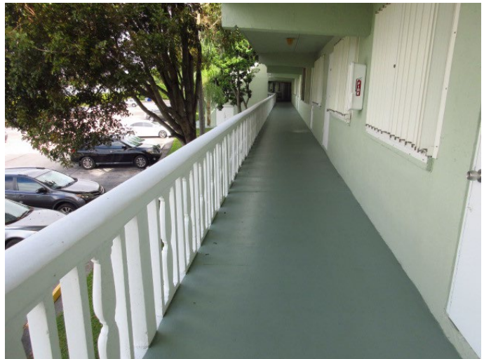
GENERAL VIEW OF ELEVATED WALKWAY
