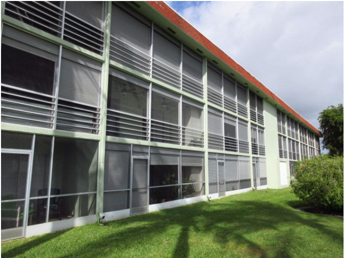
GENERAL VIEW OF BUILDING EXTERIOR FINISHES
