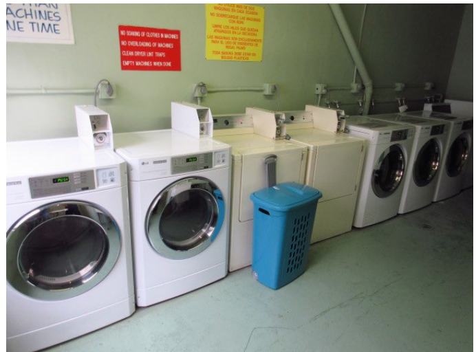
VIEW OF COMMON AREA LAUNDRY ROOM
