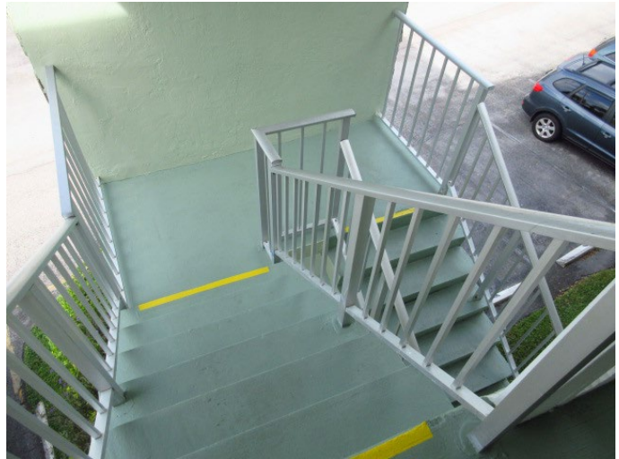
GENERAL VIEW OF EXTERIOR STAIRS
