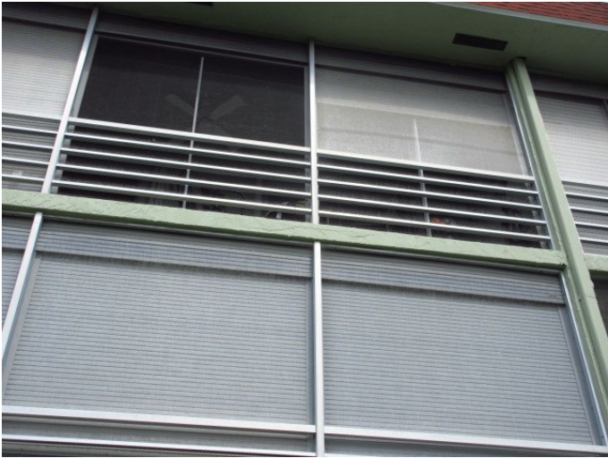
VIEW OF CRACKS AT BALCONY DECKING
