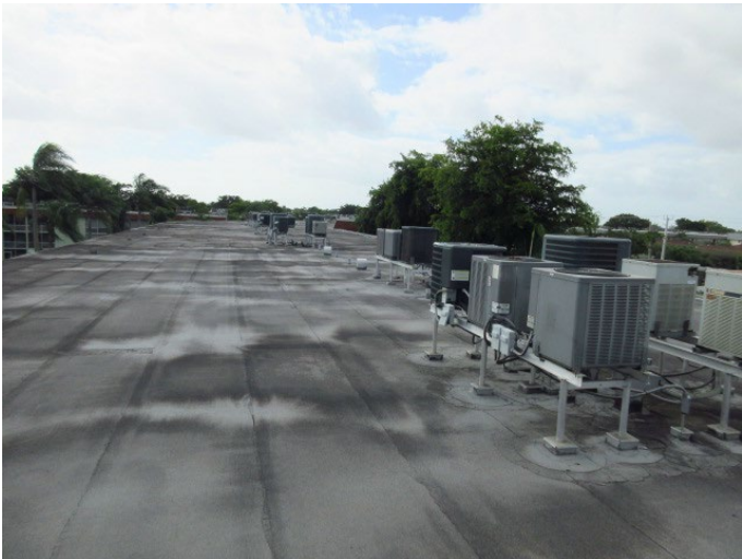
GENERAL VIEW OF ROOF COVERING
